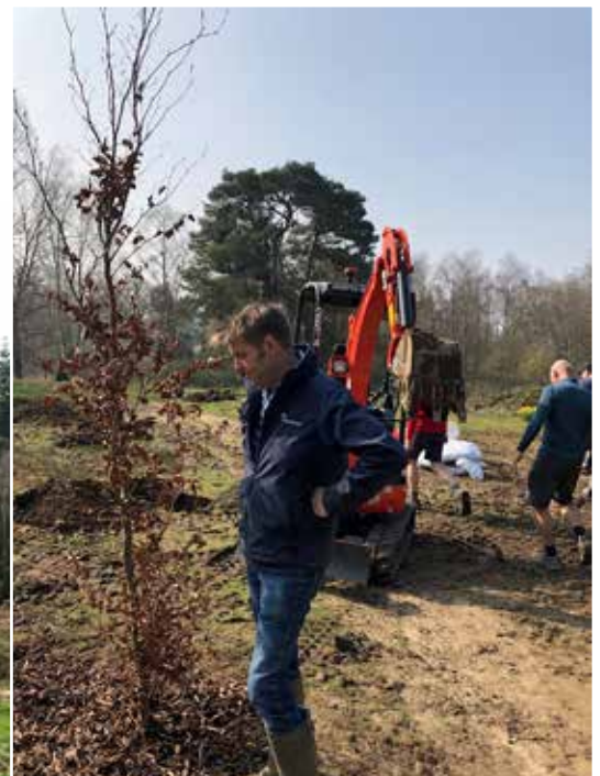
Directors of Foth, Nancy Loates-Taylor and Alex MacKinnon inspect the green bags that will water the trees.
